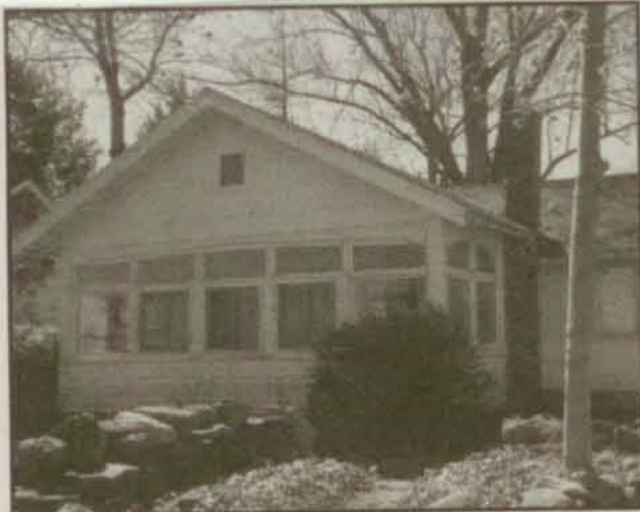
The brothers are currently reconstructing this cottage near Lake Ontario.
